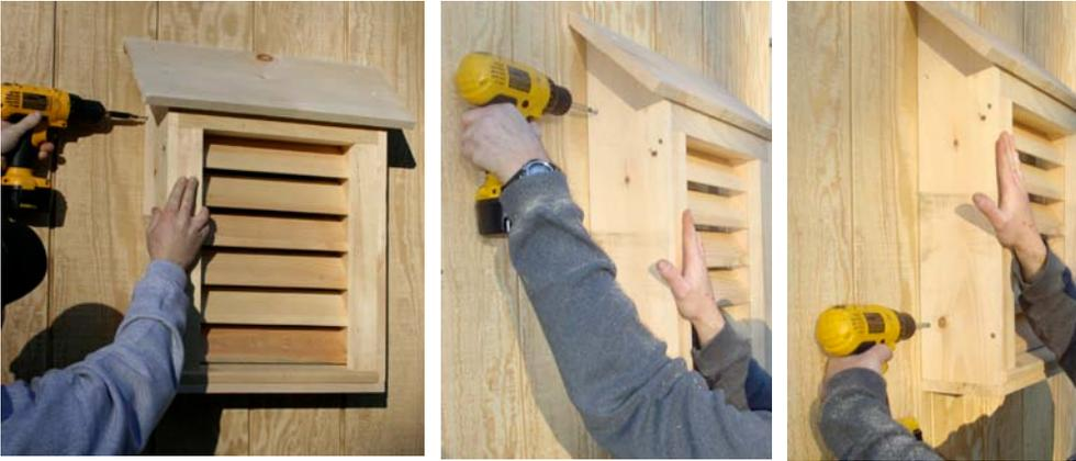
Push the Bat house hard up against the side of the house to be sure that all sides are flush against the siding. Sink screws through the pilot-holes and into the side of the gable vent as shown in the pictures above. Do this on both sides. You will use 4 screws total.
