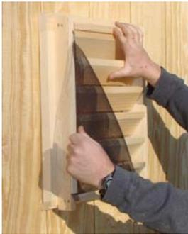
Remove Factory Bug Screen from the new Gable Vent Remove Factory Bug Screen from the new Gable Vent
