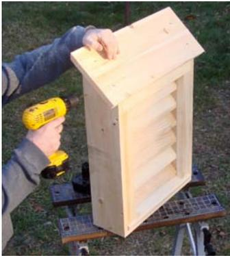
Before you go up the ladder you need to drill 4 holes in the sides of the bat house. Drill one hole on each side in the location shown above. Then drill another hole approximately 3 inches up from the bottom on both sides underneath the first holes. These will be the holes used to secure the bat house to the gable vent.
