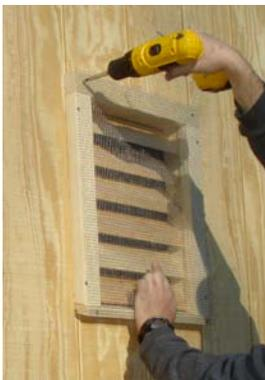
Cut the piece of 1/4" galvanized screening to fit over the entire gable vent. (the one that is installed on the side of your house)
