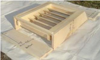
Fasten the side left and right side pieces to the side of the gable vent as shown in the picture above. Make sure that the bottom of the pieces are flush with the bottom of the vent and the front of the pieces are flush with the front of the vent as shown in picture.
